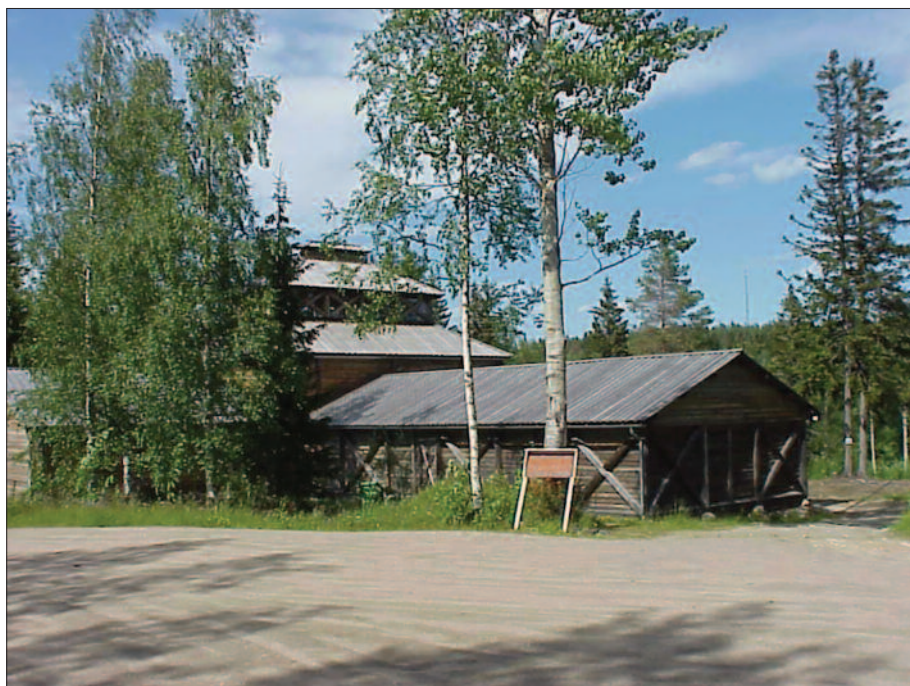
Figure 19. The original mine and its associated museum, is open during the summer months (N61° 44.52 E15° 09.40). Surrounding the museum are old shafts hidden by vegetation, all surrounded by fences to prevent accidents of nasty falls. Mining ceased in the early 1900s. Today one can take a tour deep into the mine where the cobalt ore had previously been found. When the authors took the tour, their Geiger counter was activated strongly at a level only 20 meters below the surface, attesting to the ubiquity of uranium ore which can be found in almost anywhere.
