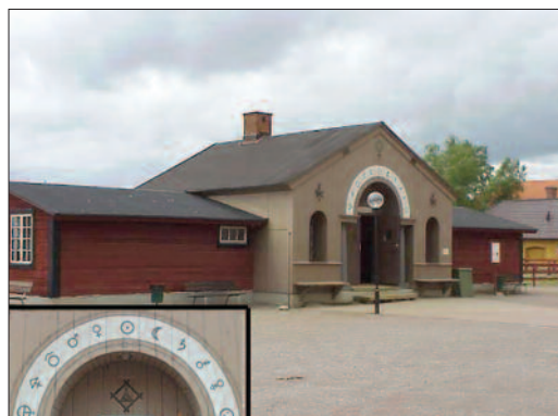
Figure 15. The entrance to the Falun Mine (N60° 36.01 E15° 36.95). The side buildings are painted with Falun Red paint (Swedish = “Falun rödfärg”), prepared by mixing water, rye flour, linseed oil, and Falun mine residues containing mostly iron oxide. Above the door are a number of alchemical symbols for various elements and salts (see inset, lower left). A splendid museum (above ground) holds great interest for visitors. Tours may be taken to the huge frigid underground (5°C); visitors must wear water-proof capes and hard hats.
