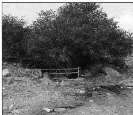
Figure 14. One of many shafts which led down to the lead mines. These shafts have not been filled in and are very dangerous to explore.
