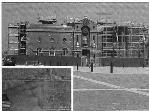
Figure 4. The Royal Military Academy Building, where the actual preparations of the barytes medication and analysis of the strontium salts were made by Cruikshank. Inset: This building can be placed during the Georgian period because of the "penny roller" style (thin recessing) of jointing between bricks.
