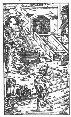
Figure 16. Smelting lead ore, from Agricola's *De Re Metallic*.
