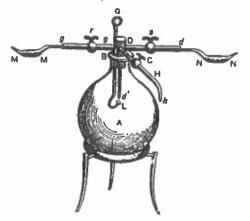
Figure 28. Lavoisier's apparatus wherein hydrogen and oxygen were sparked and reacted to form water.
